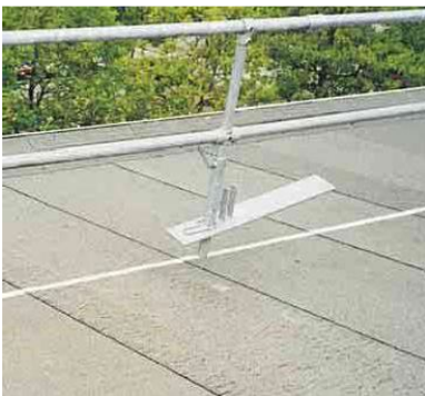
Full edge protection maintained during refurbishment and repair work
