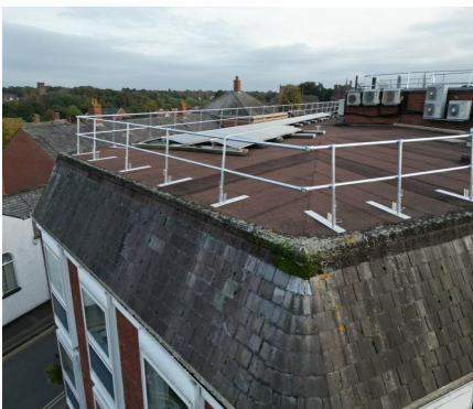
*Varying examples of completed Shorguard SG4 Edge Protections
