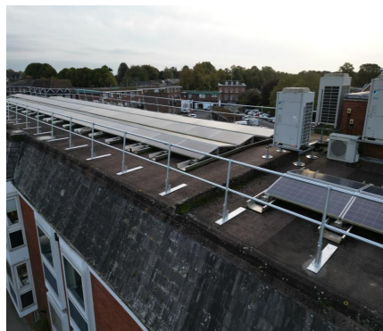
*Varying examples of completed Shorguard SG4 Edge Protections
