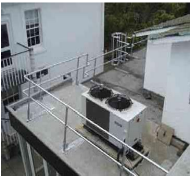
The system can be designed to accommodate various roof fixtures such as air conditioning vents
